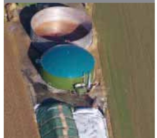
Biogas installation Biogaz installation
