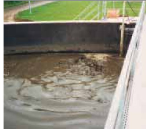
Sludge application Application de boue
