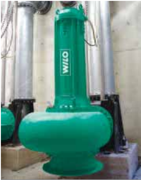
Wet sump installation Montage immergé
